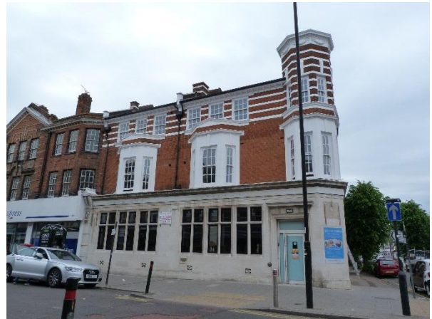
Recently Refurbished No. 150
