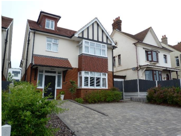
Example of a modern infill property on Ditton Court Road
