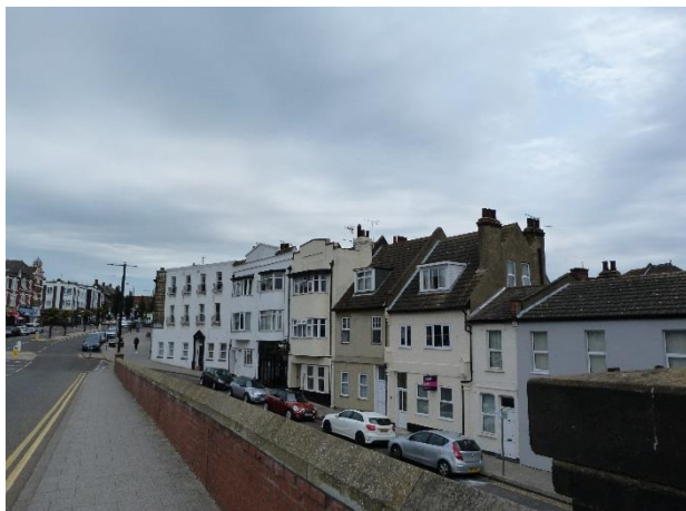
Buildings rendered and painted, with uPVC window replacements, at the southern end of Hamlet Court Road
