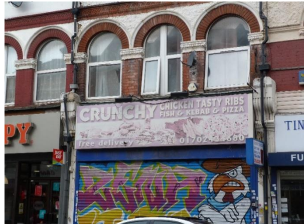
A number of inappropriate features, such as roller shutters, uPVC windows, satellite dishes and plastic downpipes, as well as an example of graffiti
