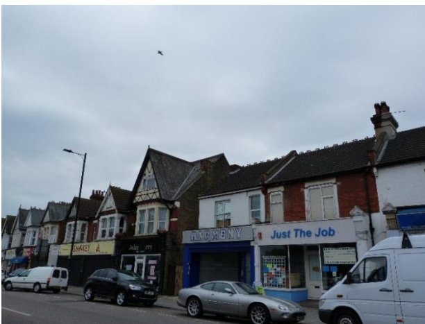
London Road lined with two storey shops
